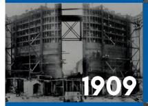
Gatun and Miraflores Locks. With a total length of over 1.9 miles, this was the largest concrete construction undertaking in the world at the time
