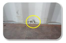
All weld seams, floor lashings and floor bolts need to be checked for sharp edges and heavy rust.
